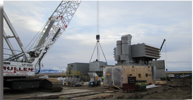
Recent construction activity near the turbine generator at the HGS site.
