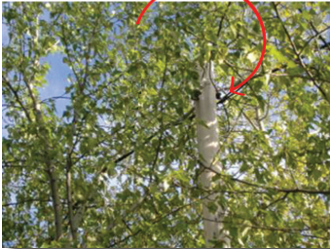
Steve's winning entry— secondary power line deflected and stressed by tree
