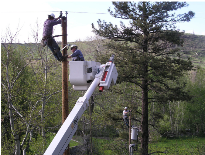
BEC Linemen Jason McDonald, Eric Elton and Gus Behrent rebuild washed out line in the Bridger Creek/Reed Point area.
